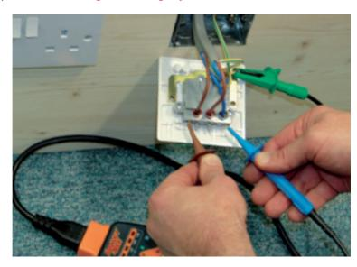
At the Socket Test stage the PDL 200A and PDL 234 also accurately measures and displays the Mains Voltage on one of the 3 LED's.
