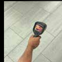
Check floorheating for leaks
